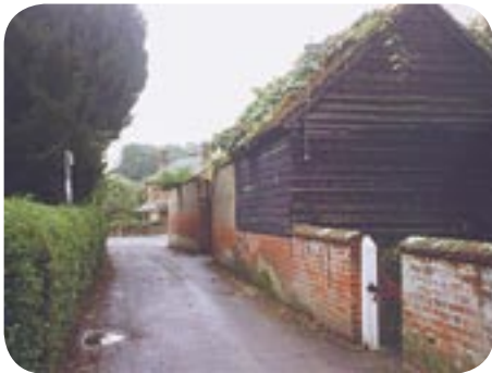
Timber clad outbuilding adjoining Church Path
