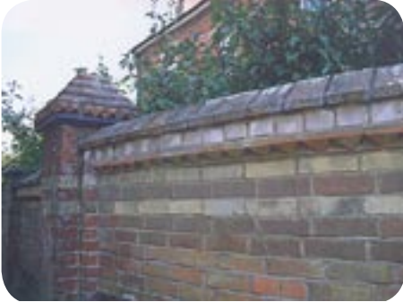
Wall detail at Springfield House
