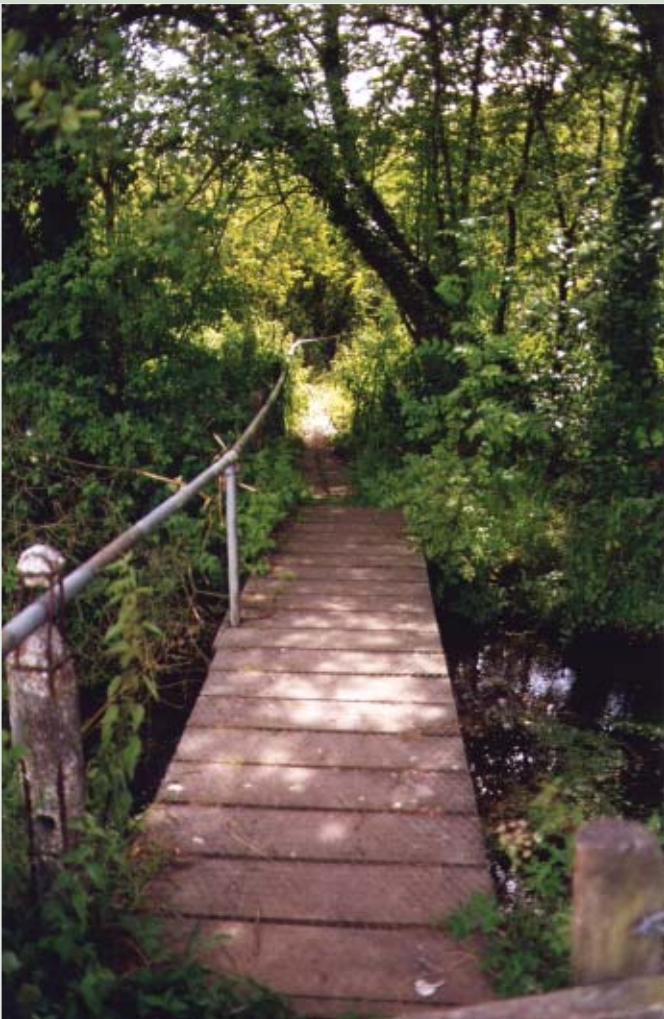
Trip-trap bridge on footpath north
