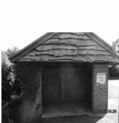
1 Cranes Rd Bus Shelter
